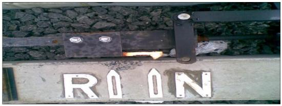
Figure D2 – Example of claw-lock signage
