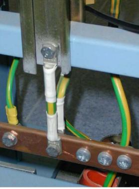
Figure C17 – Good Example of Earthing Installation
