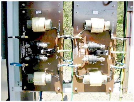
Figure C18 – Poor Example of Surge Protection Installation
