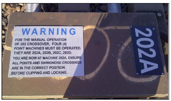
Figure D12 – Location of Points Manual Operation Warning Notice on D84M motor.
