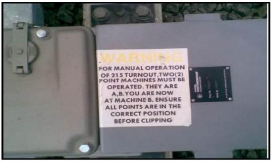
Figure D11 – Location of Points Manual Operation Warning Notice (note WARNING lettering incorrectly yellow).
