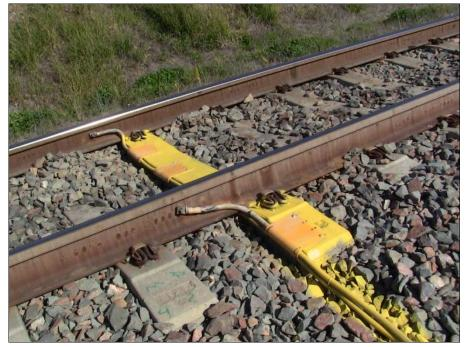
Figure 4.1 – CSEE cables protected by flat metal plates
