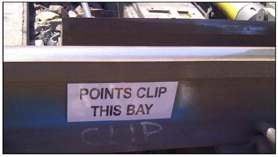
Figure D13 – Location of Points Manual Operation Warning Notice on D84M motor.
